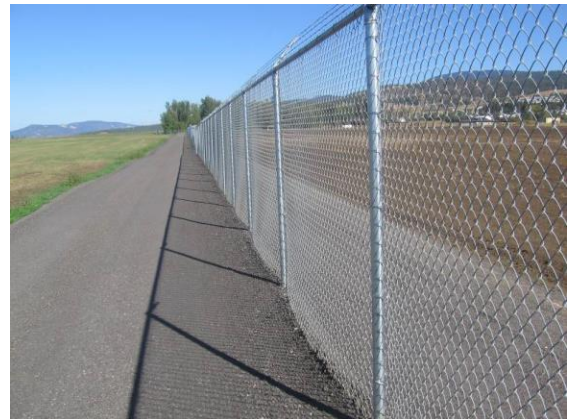
Use of asphalt tailing at fence line
